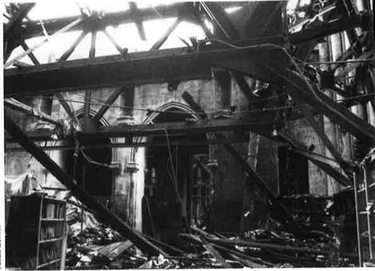
The steel beams fell to the intense heat of the five-alarm fire on the morning of December 18, 2001.
