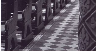
Closeups of the completed tile restoration at Central Synagogue.
